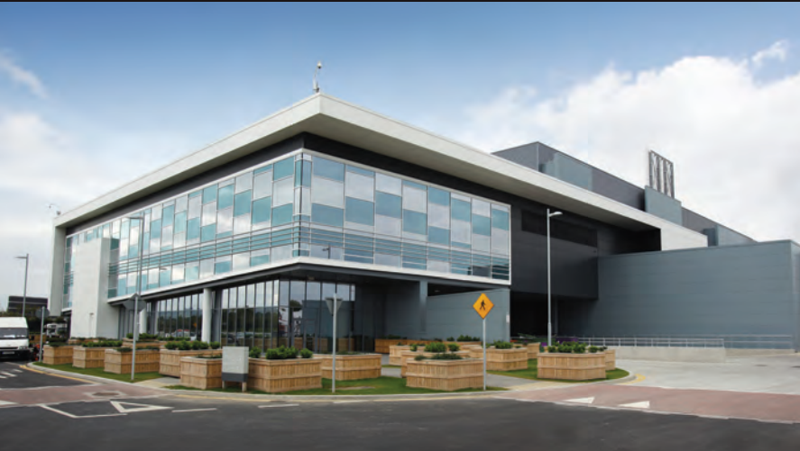
Microsoft 29.4MW Data Centre, Dublin
