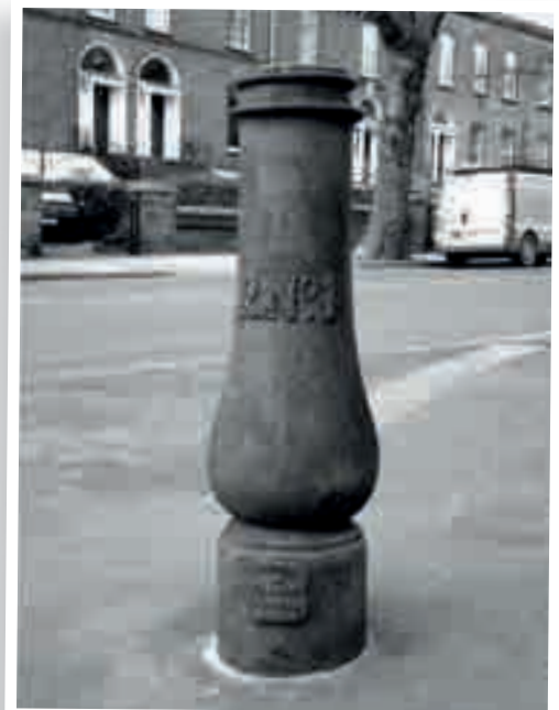
Above: A relic of Dublin's early sewerage system: a cast iron sewer vent on a footpath in Leeson Park, manufactured by the famous foundry of Tonge and Taggart, Dublin.
