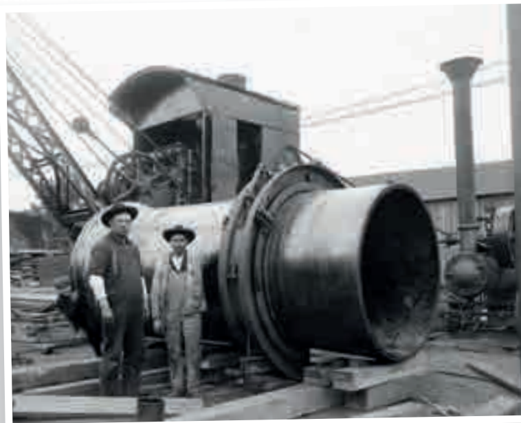
Above: The cutting edge of technology circa 1900: operatives cutting a 48-inch cast iron pipe in Philadelphia, a city noted for its advanced plumbing and sewerage system. When Harry O'Neil returned to Dublin from America he brought with him his knowledge of the most innovative skills in the design and installation of sanitary piping systems.
