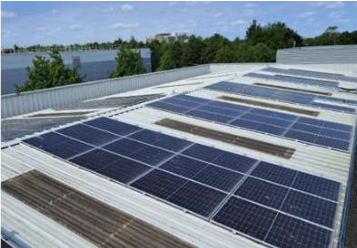
70 kWp solar PV system at our Damastown facility.
