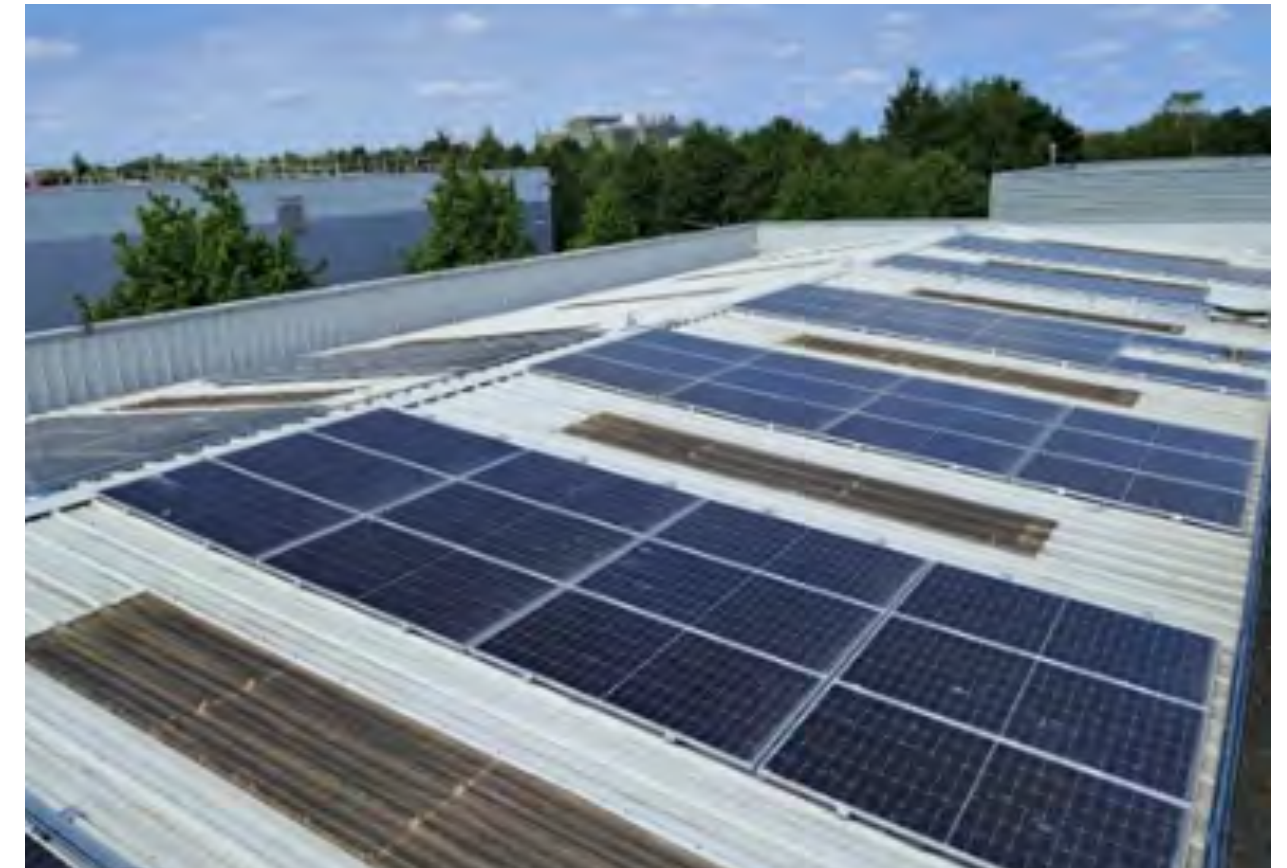
70 kWp solar PV system at our Damastown facility.
